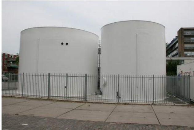
FIGUUR 2.4 MBR TANK (L) EN VERGISTER (R)
